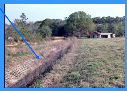
Number 23. Install water control system -- Control water on land by means of surface or sub-surface drains and structures. Use where the rooting zone is thin or thick due to a seasonally or permanently high water table.
